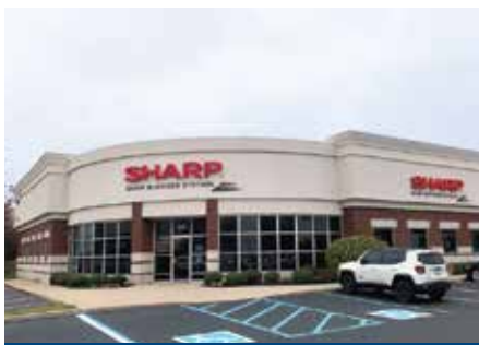
86th Street Business Center Indianapolis, IN
