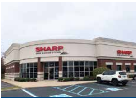
86th Street Business Center Indianapolis, IN
