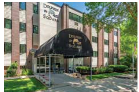
Dolphin Square Apartments Wauwatosa, WI
