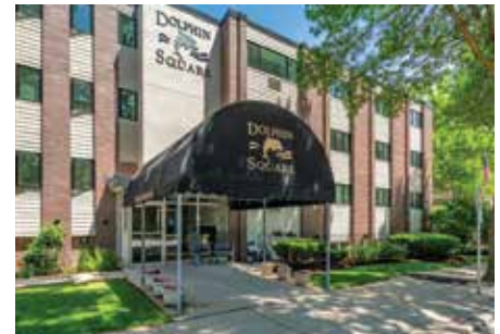
Dolphin Square Apartments Wauwatosa, WI
